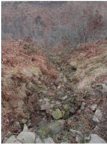
I17 – J2.6. An example of a dry ditch.
