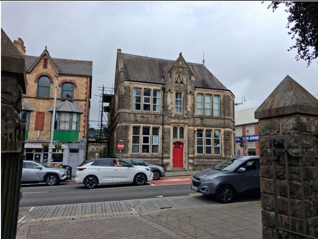
Plate 70: West view towards North Company Offices (A174) from gateway to Church of St David (A57) within Maesteg Conservation Area (A29)
