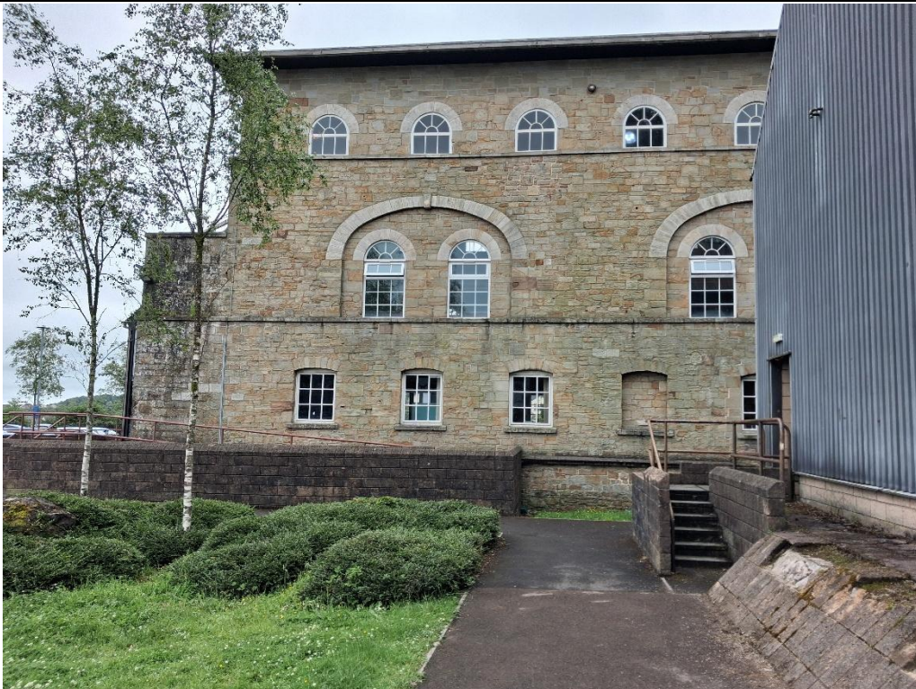
Plate 60: Northern elevation of former engine house, Grade II listed Maesteg Sports Centre (A36)
