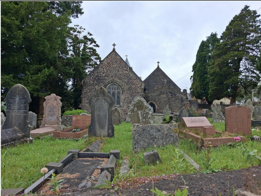
Plate 54: Eastern elevation of Grade I listed Church of St David, Bettws (A32) within immediate setting of churchyard
