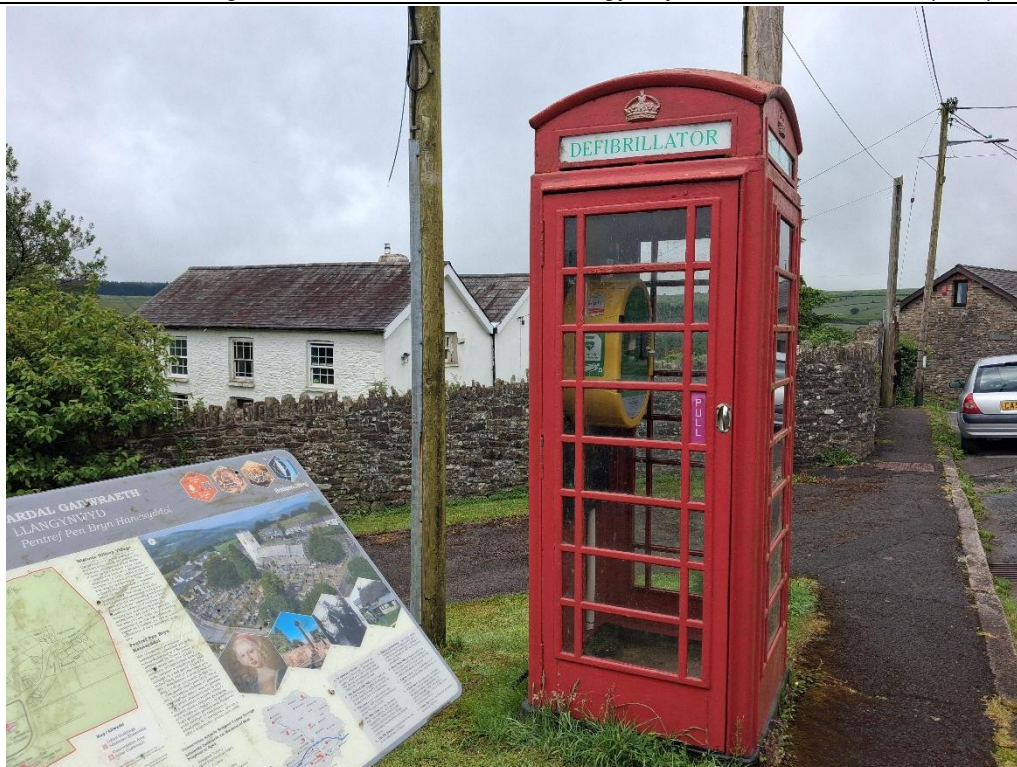
Plate 50: Heritage information board adjacent to Grade II listed telephone box (A172) within Llangynwyd Conservation Area (A30)
