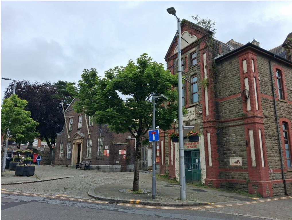
Plate 65: Northeast view of Colonel North Memorial Hall (A58) within Maesteg Conservation Area (A29)
