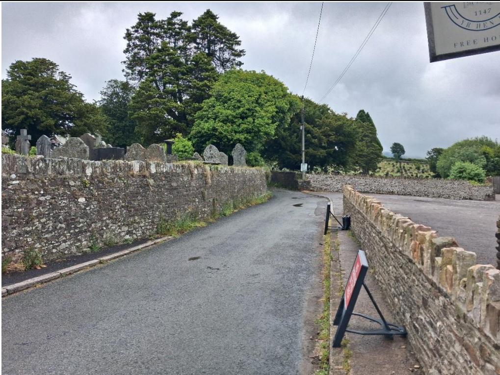
Plate 48: East view of Grade II listed churchyard walls (A84) within Llangynwyd Conservation Area (A30)
