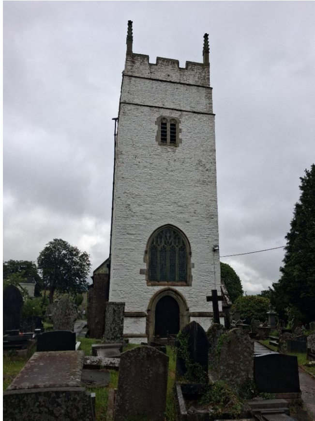
Plate 46: Western elevation of Grade II* listed Church of St Cynwyd (A33) within Llangynwyd Conservation Area (A30)
