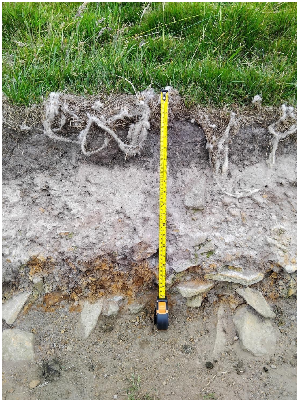
Plate 11B.7 – Mineral profile at exposed soil margin location S4 (Southern Array). Topsoil was classed soft pale grey slightly organic slightly silty clay with rootlets, over upper subsoils comprising soft dark grey clayey silt with orangish brown mottles with lower subsoil characterised by soft orangish brown slightly gravelly clayey silt. Gravel content in subsoils increased with depth, of primarily medium sized sandstone fragments that are subangular in shape. NGR: SS 89311 89907.
